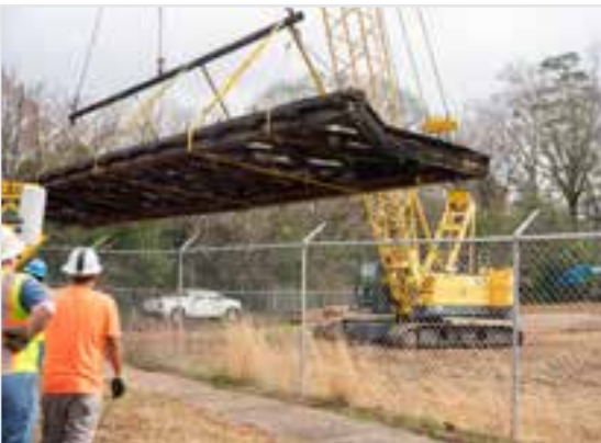
Moving one of King's bridges from its original location to its new home next to King's place of rest in Mulberry Street Cemetery.
