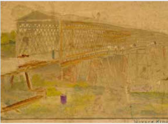
Barely visible in the lower right hand side of this image, Horace King stands in front of Glass Road Bridge, one of King's many local bridge projects.
